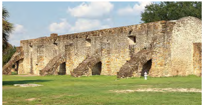
MISSION SAN JOSE BUTTRESSES AND MASONRY
